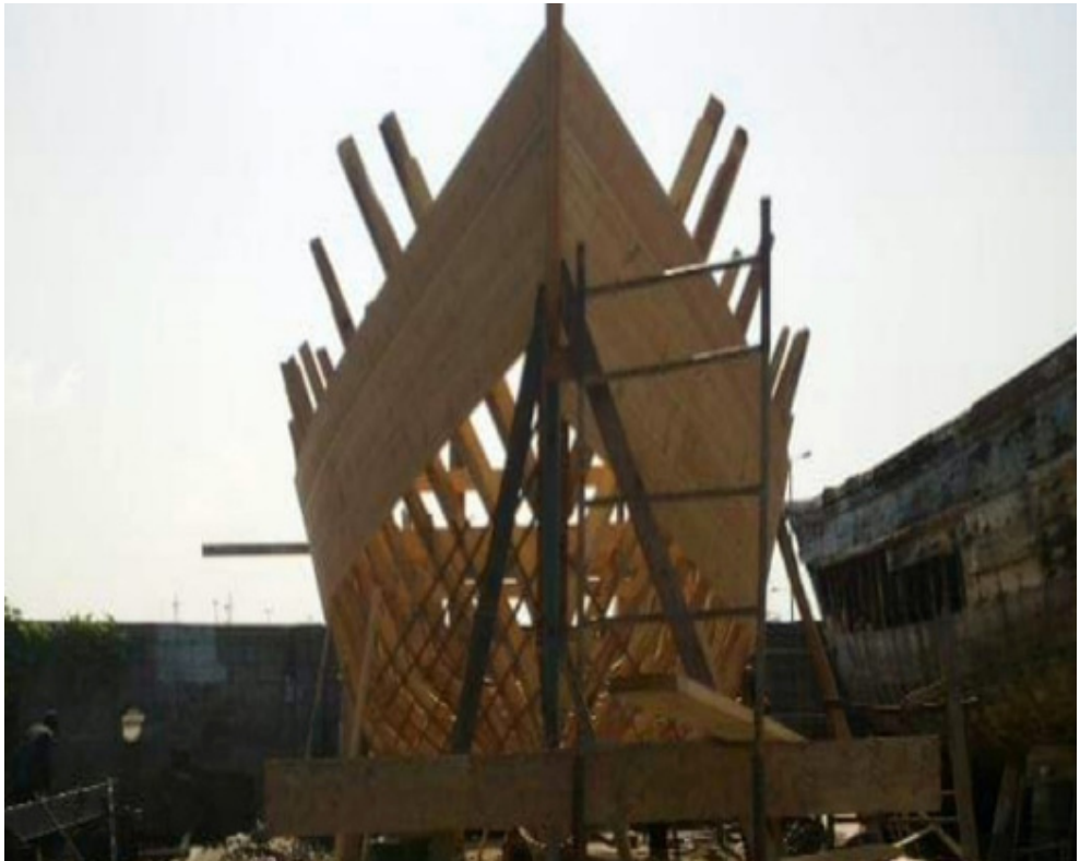
Ship under Construction on the Coast of Jazan
