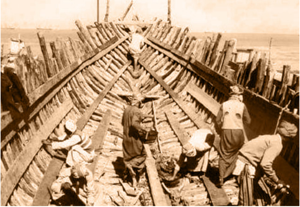
Stage 4: Placing the Keel in the Ship
