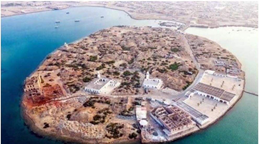
Recent Photo of Suakin after Restoration Work on the City's Buildings
