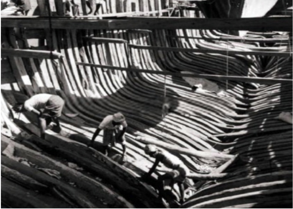
Fixing the ribs of a wooden ship, Shipbuilding Center, Al-Mualla, Aden, 1950.
