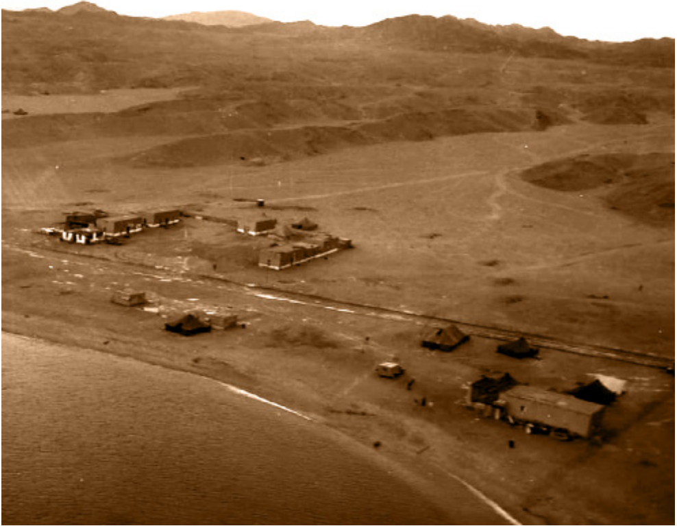
An aerial photograph of Umm al-Rashrash taken by the Rothenberg brothers in late 1948.
